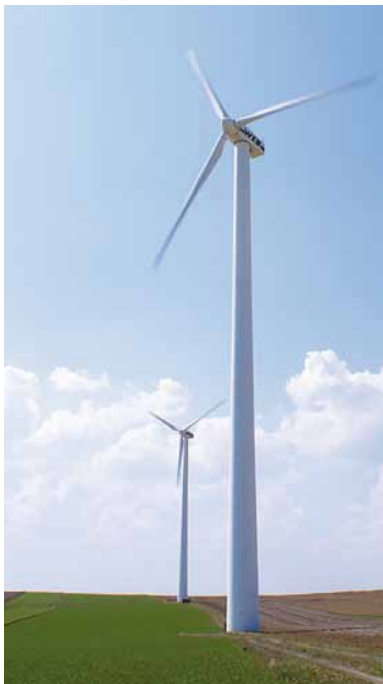
Oberstrahlbach wind park: One of WEB Windenergie AG's first sites (plant numbers 5, 6 and 7).
